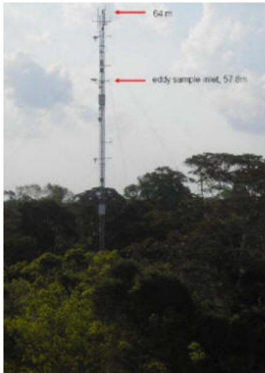
Figure 2. Tower measurements started in April, 2001 and continued until the tower was destroyed when a falling tree hit the guy wires in January 2006.
