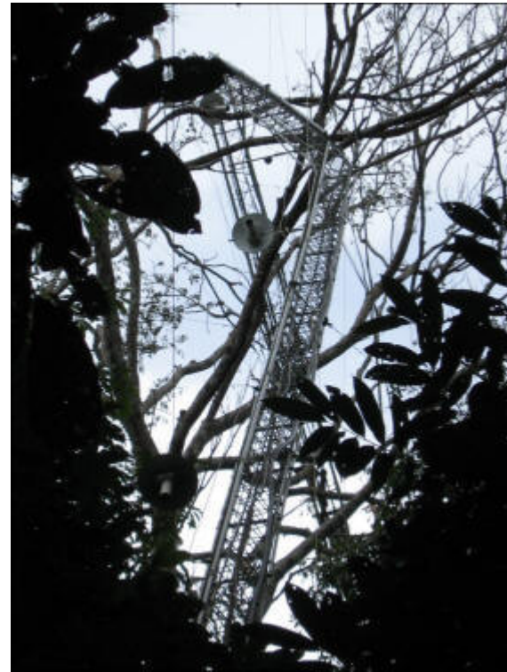
Figure 2. Tower measurements started in April, 2001 and continued until the tower was destroyed when a falling tree hit the guy wires in January 2006.
